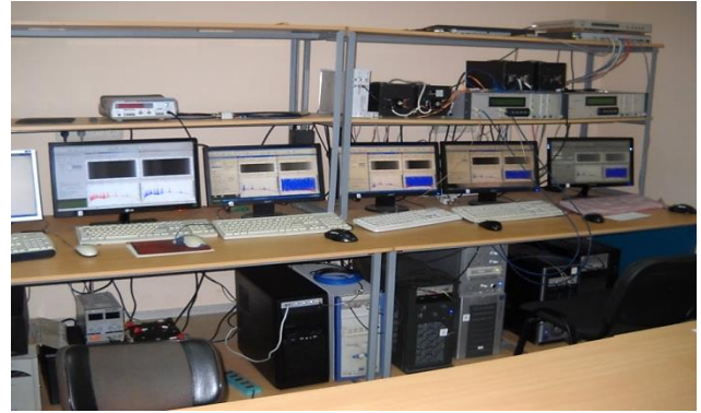
Figure 3: The UTR-2 control center with new-generation back-end facilities
